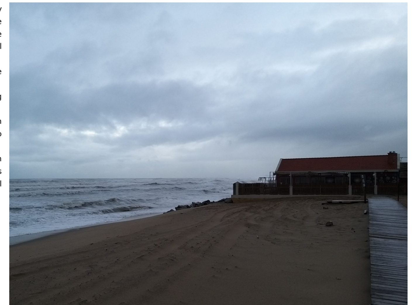
Figure 2: Beach restaurant protected by a sea wall, but still at risk
